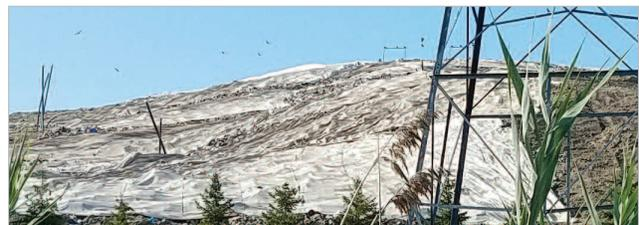
In this photo you can see how rather than soil for cover, Waste Management uses an approved “fabrisoil” to cover areas where we will be going back to work the next day.
