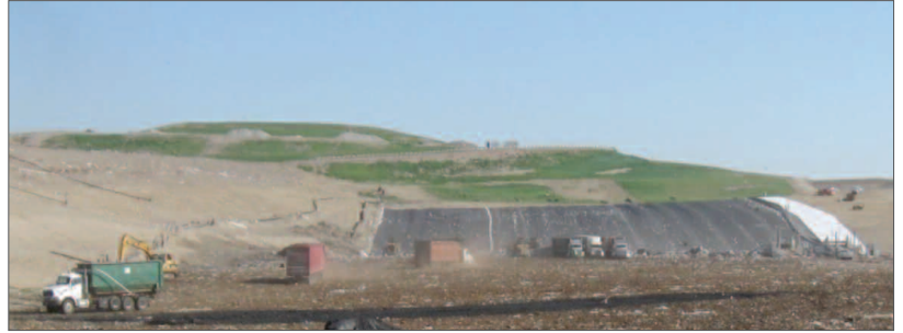
Facing north - the sidewall liner of Cell 22
